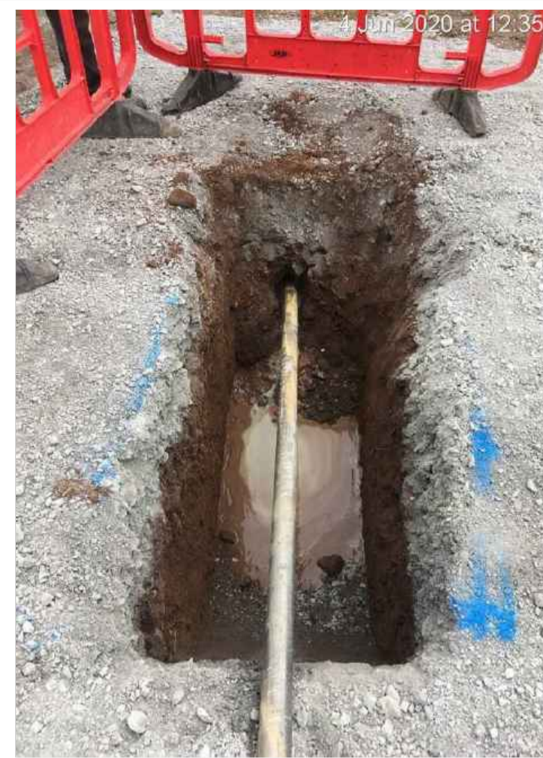
Image 3 | Typical Launch Pit
